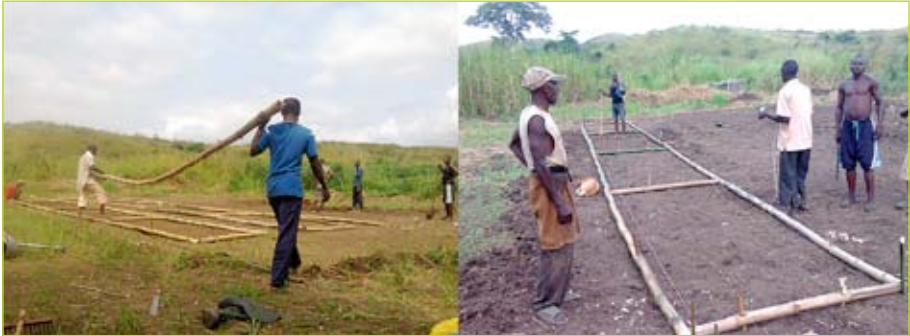
Bamboos installation and fixing with stakes, J. Scholle, GRET, DRC, 2014.
